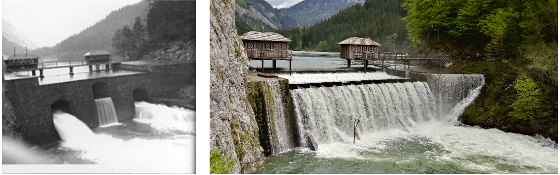
Figure 2: The Prescenyklause 1931 (left) and today (right).
